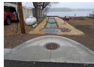
Stormwater Project on Lake Sandy Sherburne SWCD
