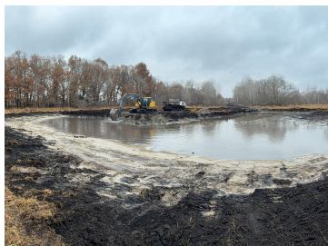
Cartwright Phase 2 Wetland Restoration Isanti SWCD
