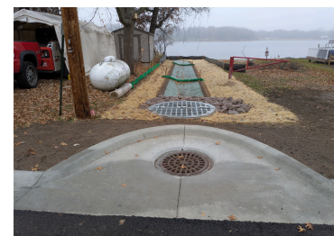
Stormwater Project on Lake Sandy Sherburne SWCD
