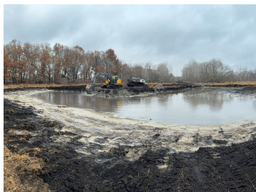
Cartwright Phase 2 Wetland Restoration Isanti SWCD
