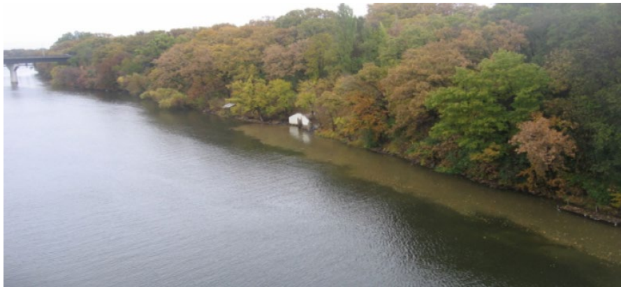
Figure 1. Drainage coming from the 96-inch outfall in NE St. Cloud. This is from an approximate one-inch rainfall event.
