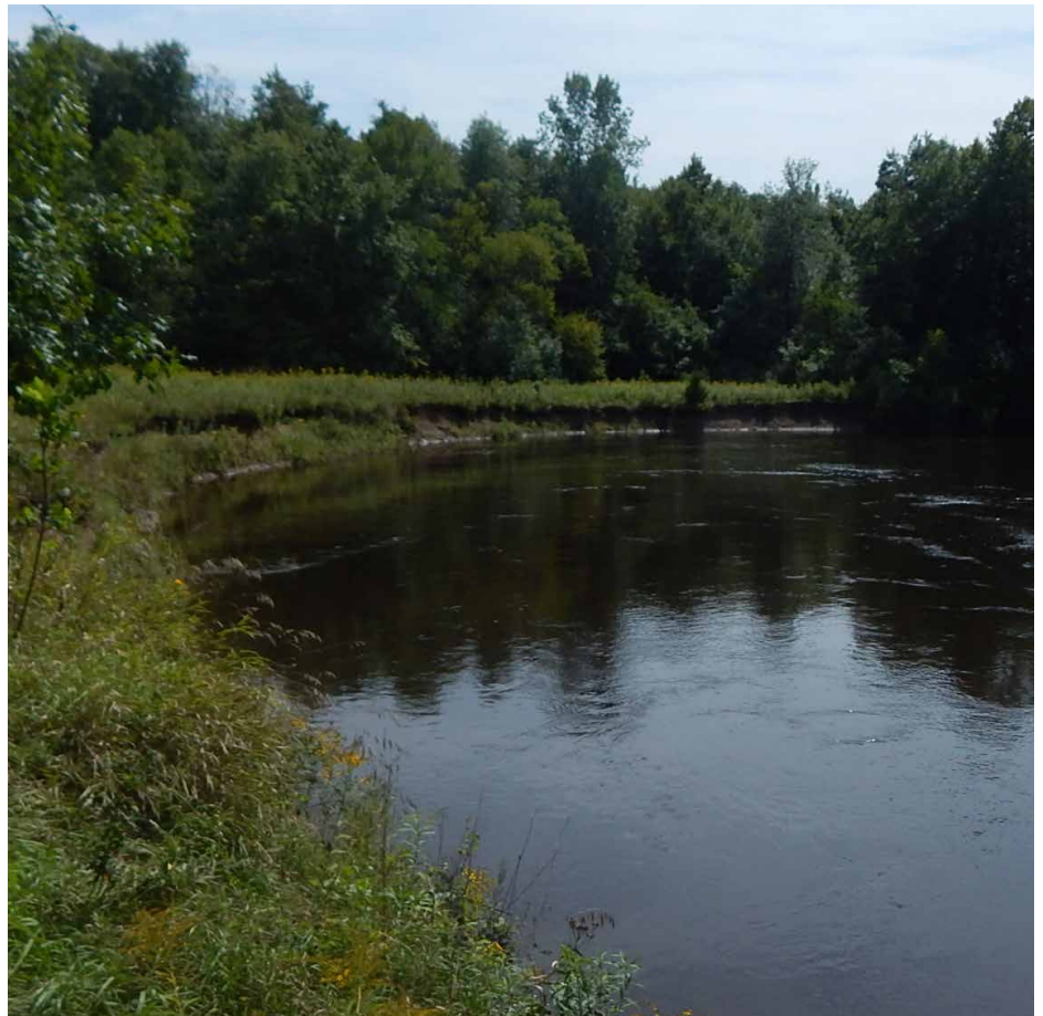
► Figure 3.1: Bank erosion on the Rum River, image courtesy of the Sherburne County SWCD
